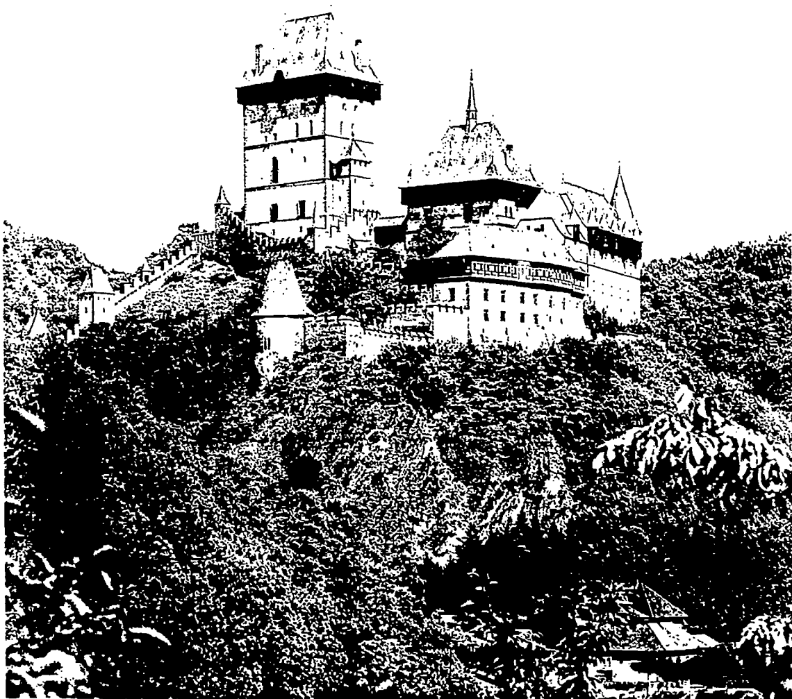
3. Karlštejn Castle. Holy Cross Chapel top floor, highest tower. 14th century.
