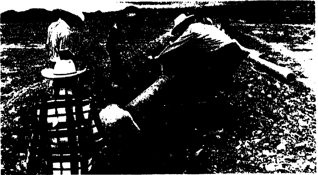
All ejidatarios participating in the project, and many of the older boys, helped to build the irrigation system.
