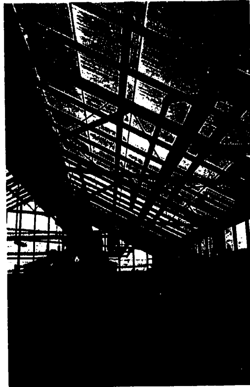
Figure 2.9 Typical even-span construction showing a purlin running the length of the greenhouse, supporting the sash bars and connecting the trusses
