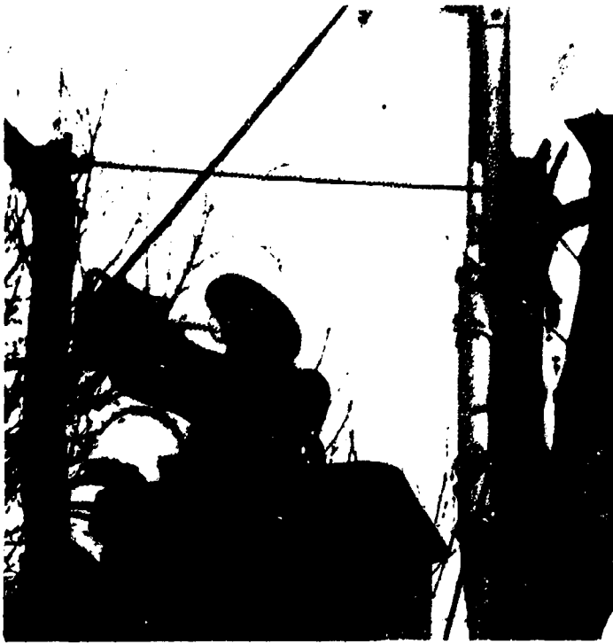
FIG. 7.4. Proper positioning of the booms is critical when removing large limbs.
