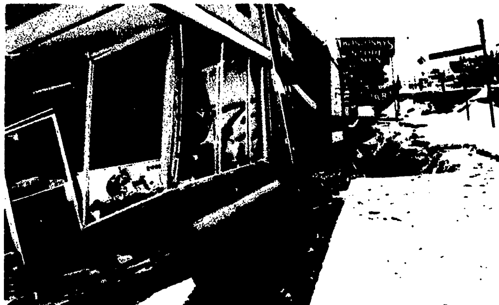
Damage caused by earthquake.
