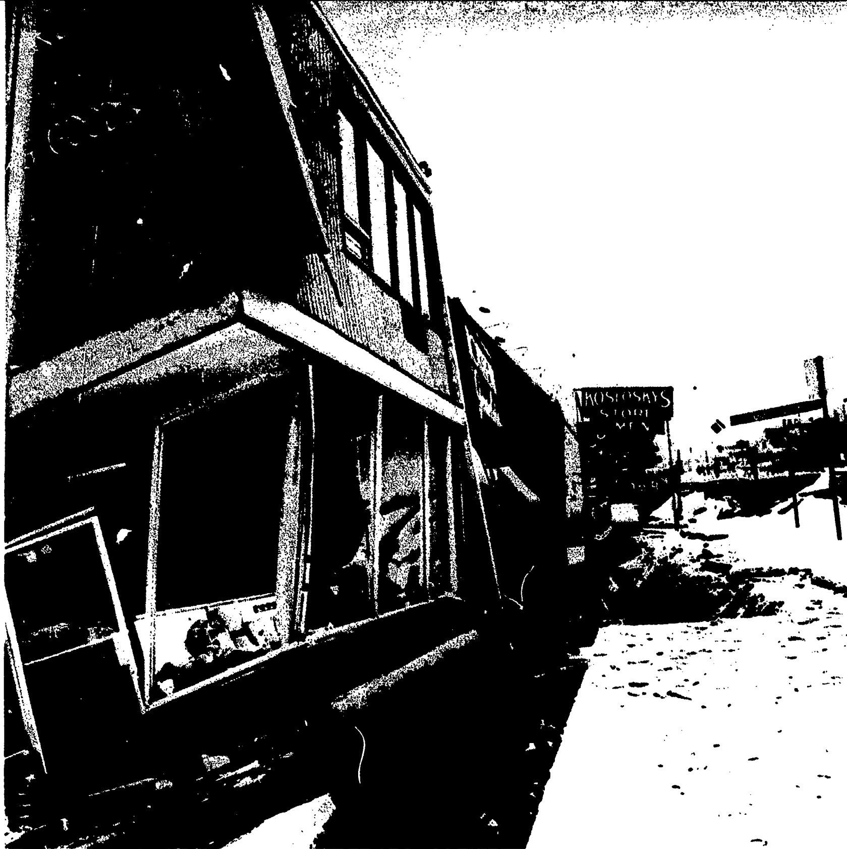
Photo left: The earthquake of 1964 caused the greatest damage in this downtown business section of Anchorage, Alaska.
