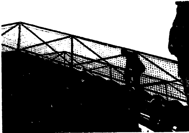
FIGURE 9. Many shapes are built from smaller ones. The reinforcing beams in a bridge illustrate how repeated patterns are used in engineering and architecture, as in nature, to form a whole out of parts.
