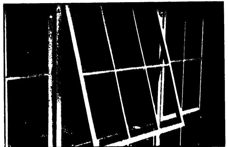
Figure 10-A. Multi-Paned Factory Window
