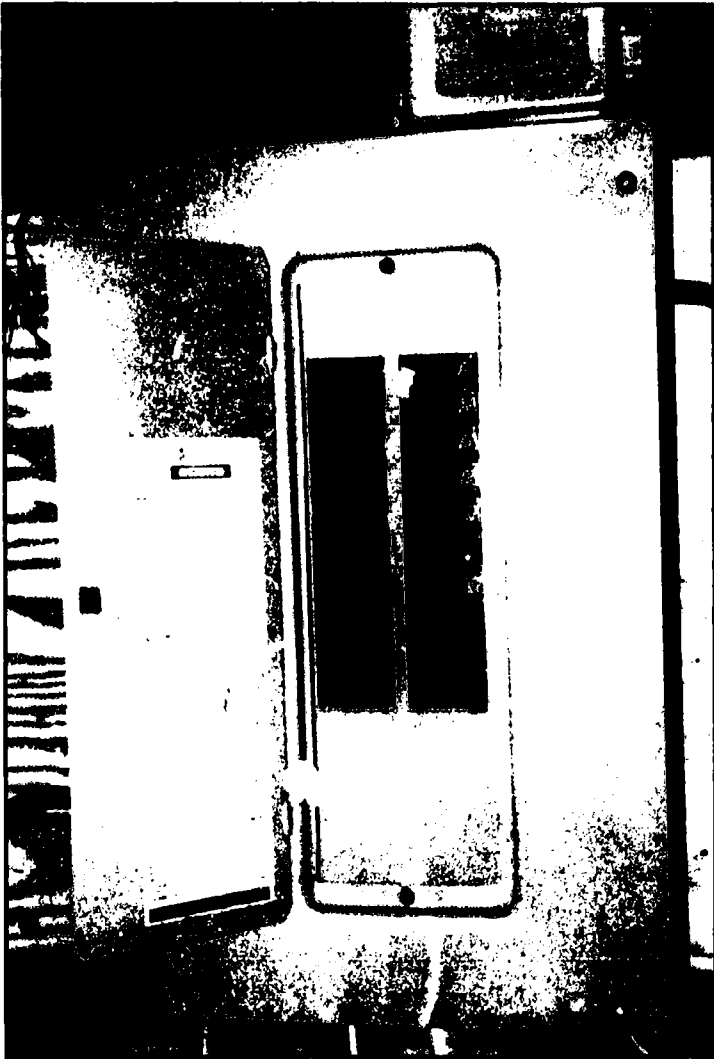
Figure 31. Circuit Breaker Box
