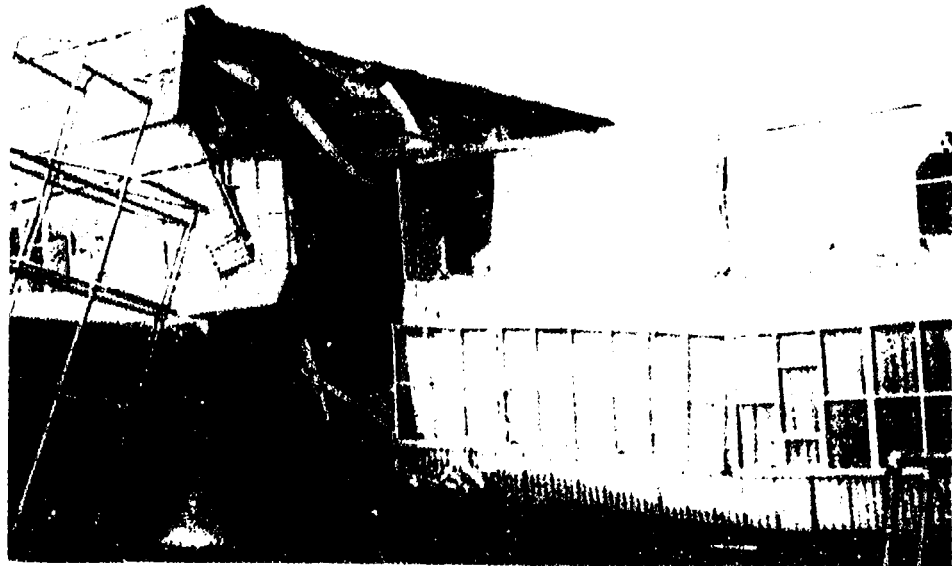
FIGURE 27 Government Hill School in Anchorage after 1964 earthquake.
