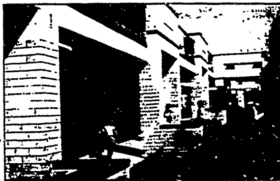
Prefabricated construction allows this school to be moved to another site if enrollment changes. Photo courtesy of Thomas Clark Associates.
