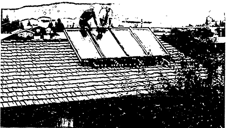
In the energy conscious era of the 1970s, NASA's operational experience found many new applications. This prototype water heater, warmed by solar cells, was installed on a home in Idaho.
