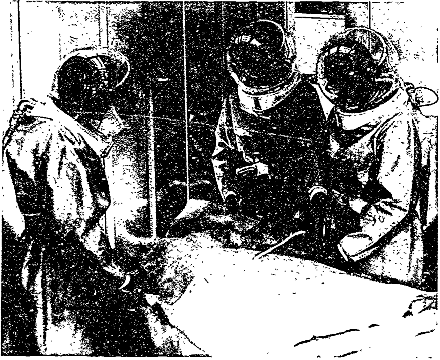
Laminar flow clean room and special clothing used at St. Luke's Hospital, Denver, in 1972 to lower risk of infection in hip joint replacements and other surgical procedures. Both the room and the clothing were based on space program experience and were developed under NASA contract by the Martin-Marietta Corporation.
