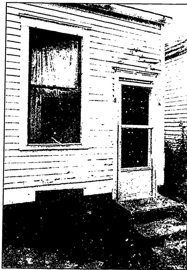
The kitchen and basement windows are broken at Hazel Summers' home. The screen door, which has no screen inserts, is not attached to the house. The triangle imprint above the door shows where the back porch roof was attached before it fell during Ms. Summers' tenancy.
