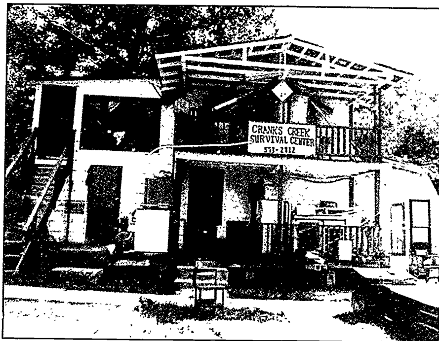
The Cranks Creek Survival Center in Harlan County, Kentucky, brimming over with recent donations.
