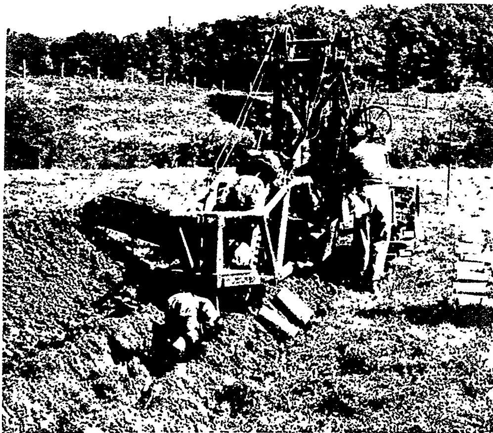
Figure 160. —Wheel-trenching machine in operation. The man at the wheel is controlling the depth of the trench by sighting over the target. The man in the trench is putting the tile in place.
