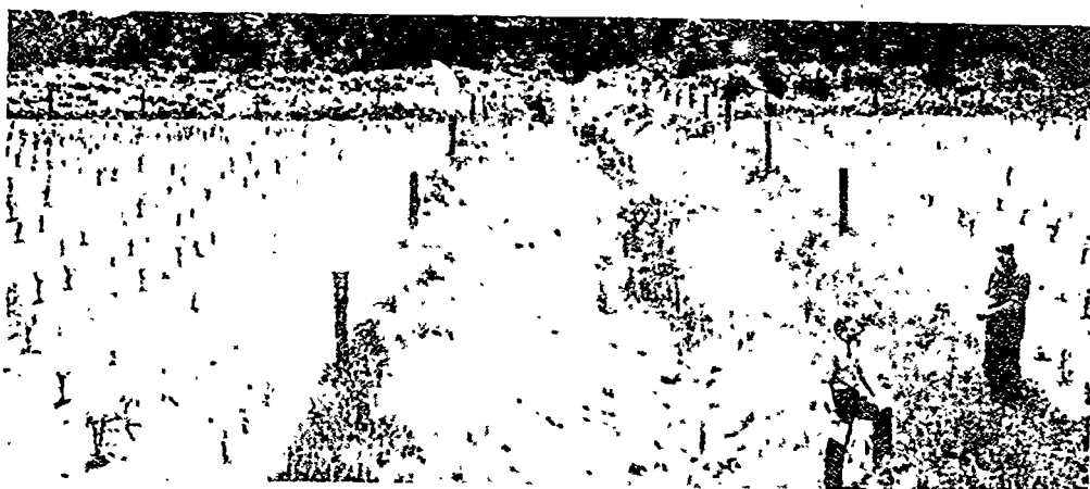
Figure 149.—V-shaped collecting ditch with the banks seeded to lovegrass.
