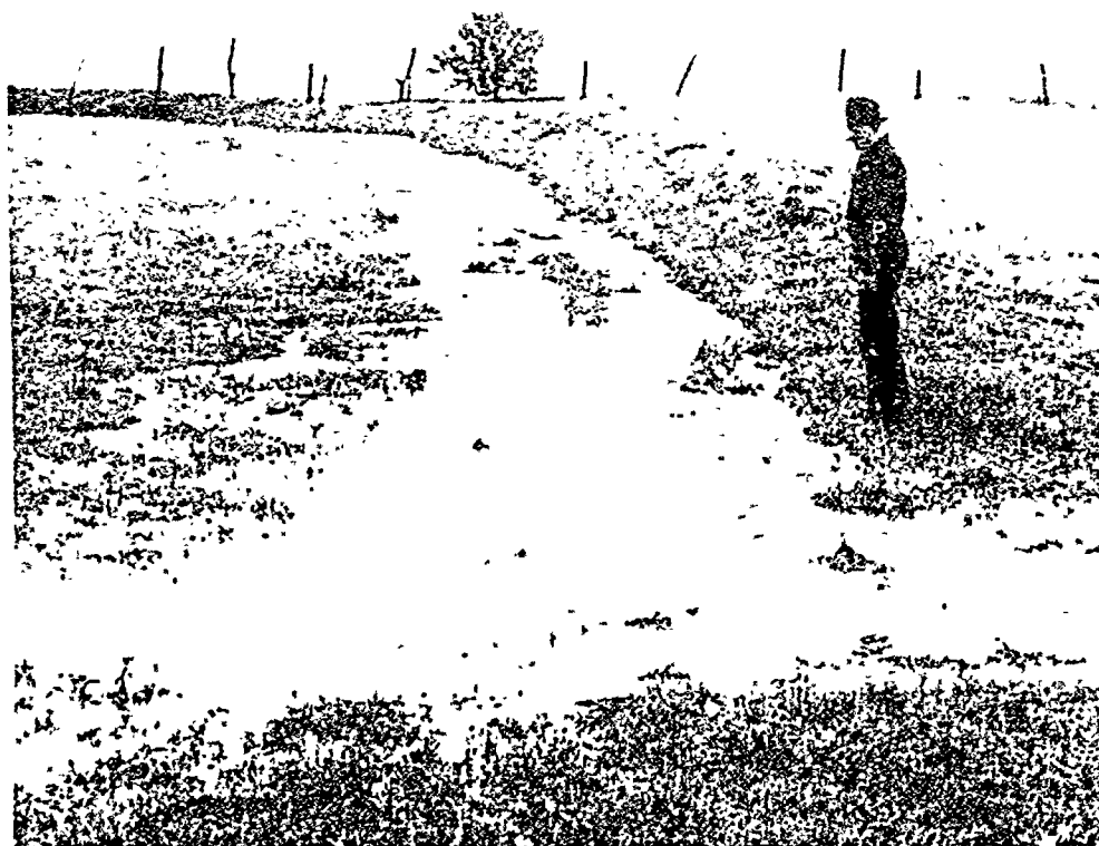
Figure 89. —A terrace discharge on pasture sod. The water spreads as it leaves the terrace channel. Much of it will be absorbed and stored in the soil.
