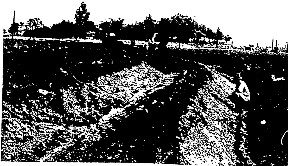
Figure 93. —Terrace construction with a plow and V-drag. It requires considerable work to construct satisfactory terraces with this type of equipment.
