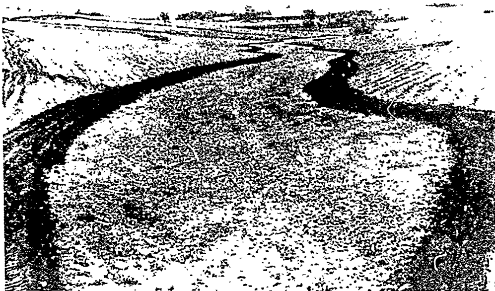
Figure 88. —Ridges along the sides protect this newly seeded meadow-strip outlet. Terraces will be constructed when the sod is well established.
