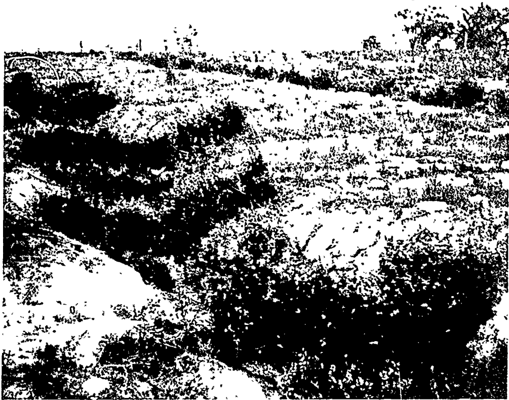
Figure 62.—Shrub checks in a small gully. Note the close spacing of the checks.
