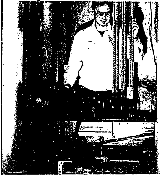
An elevator inspector checks the cables carefully.
