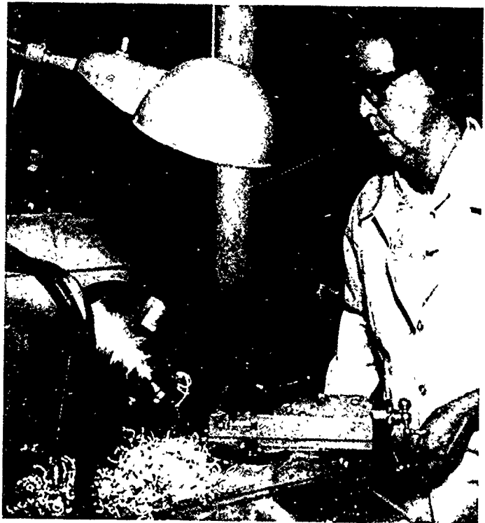
This machinist is turning a part on a metal-cutting lathe.
