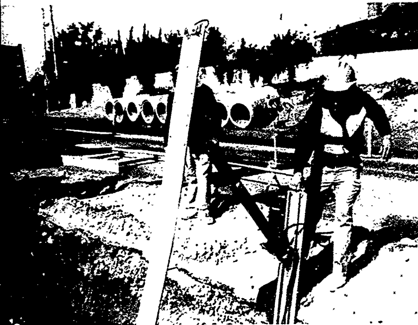
This construction worker is helping to set large sewer tile.
