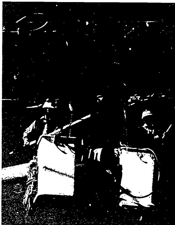
High voltage linemen often work in crane buckets.
