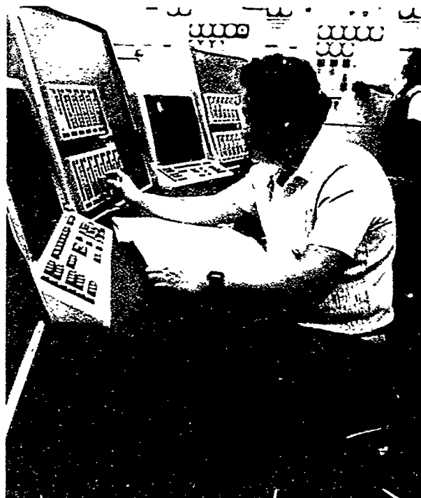
This switchboard distributes the output of a biomass electric generator.
