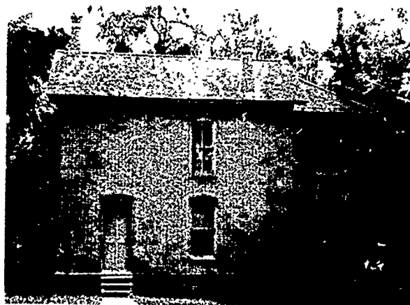
The kitchen building, which includes a brick oven and a fireplace, warmed Bailly's sickbed as he awaited his death in 1835.
