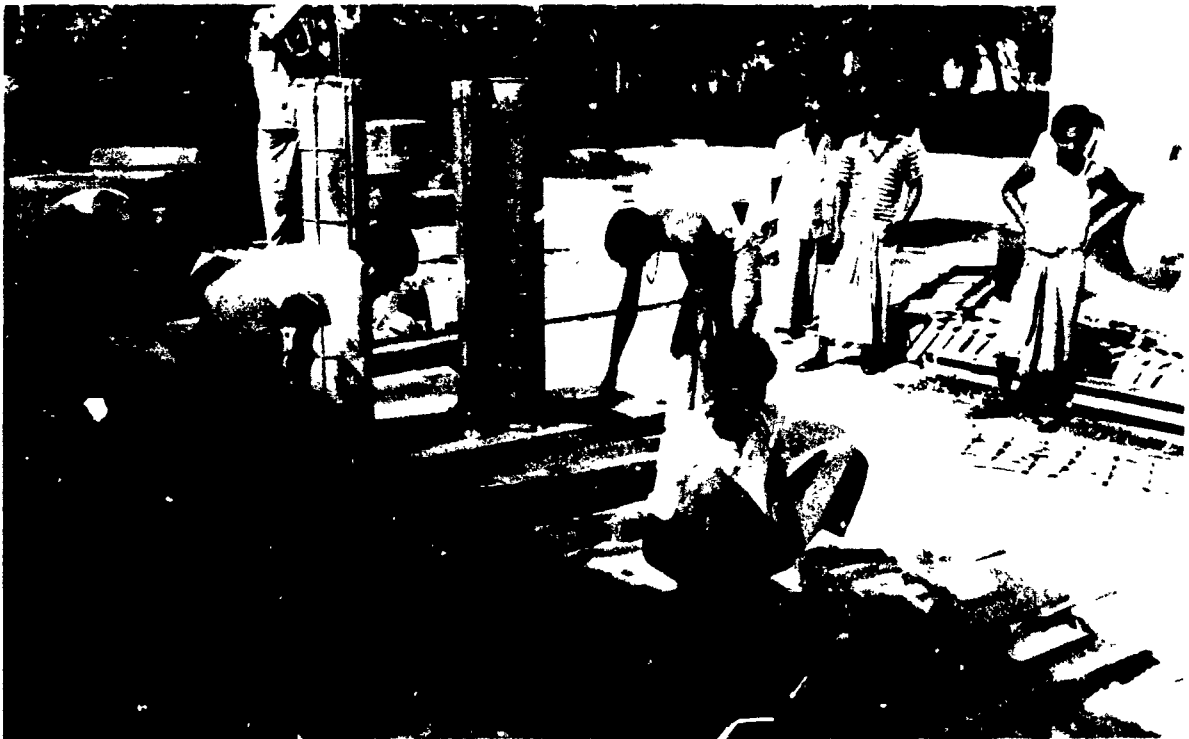
Figure 18. Removing forms from precast RCC elements. Two workmen are lifting the angle-iron frame from the wall panel while the man in the foreground is removing the louvre forms.
