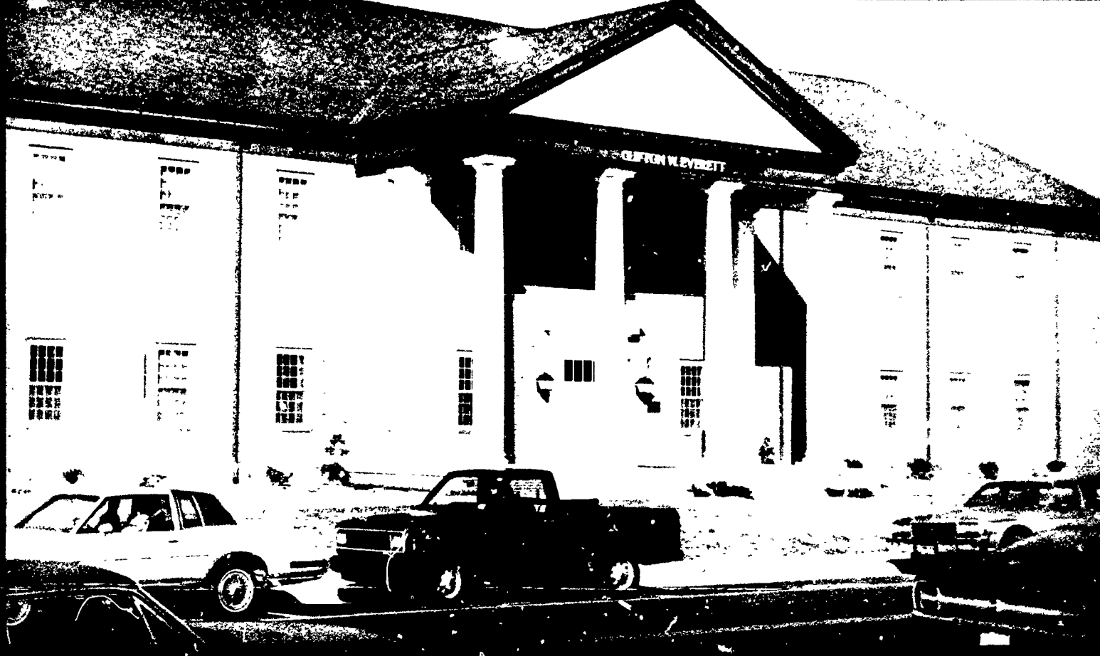
Clifton W. Everett Building Pitt Community College
