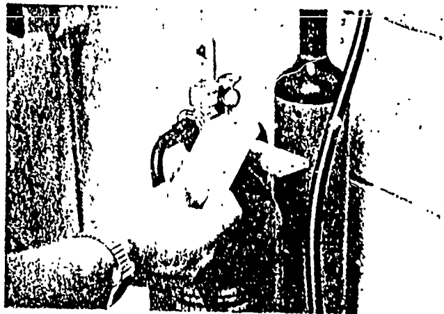
FIGURE 80. A fire extinguisher must be inspected regularly and be fully charged.
