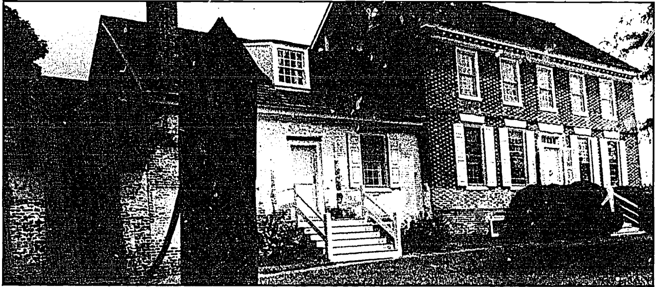
John Dickinson's plantation in rural Dover, Delaware, is the focus of extensive archeological and archival research leading toward the restoration of the grounds and outbuildings. Photograph courtesy of the Division of Historical and Cultural Affairs, State of Delaware.
