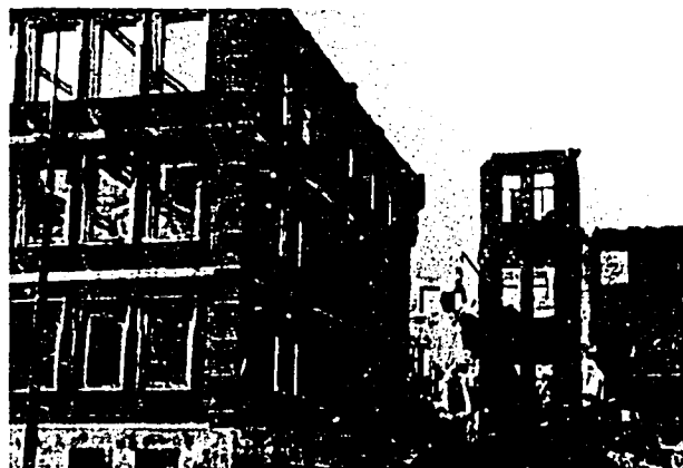
These photographs show a school building in Schwandorf, near Amberg, which was destroyed in a bombing the day after the Benzels left it — with a loss of 260 lives, all refugees. The Benzels had been housed on the third floor of the building pictured in both photographs.
