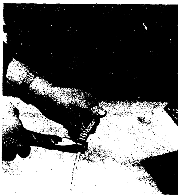
Figure 10.22. Pliers are used to wrap the strands of the dead end cable.
