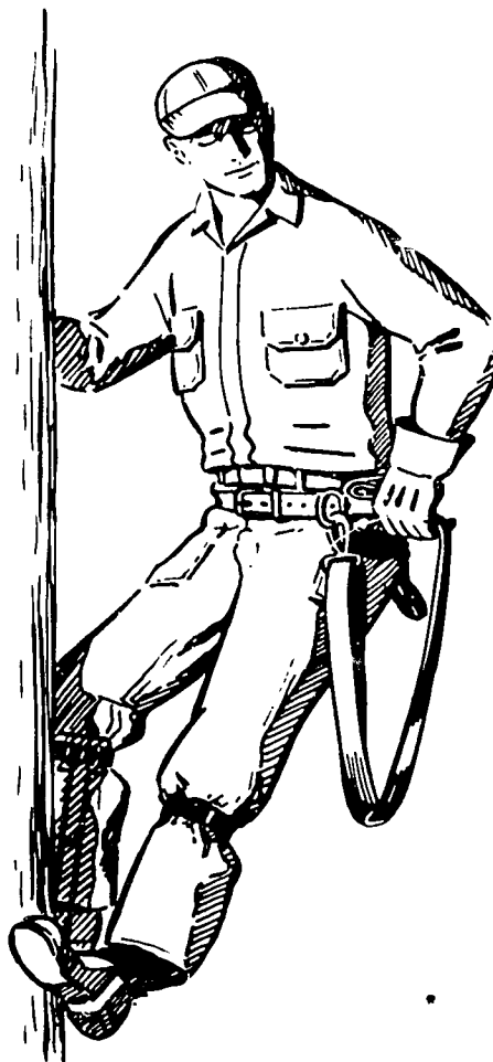
Figure 2-27. Unhooking safety strap.
