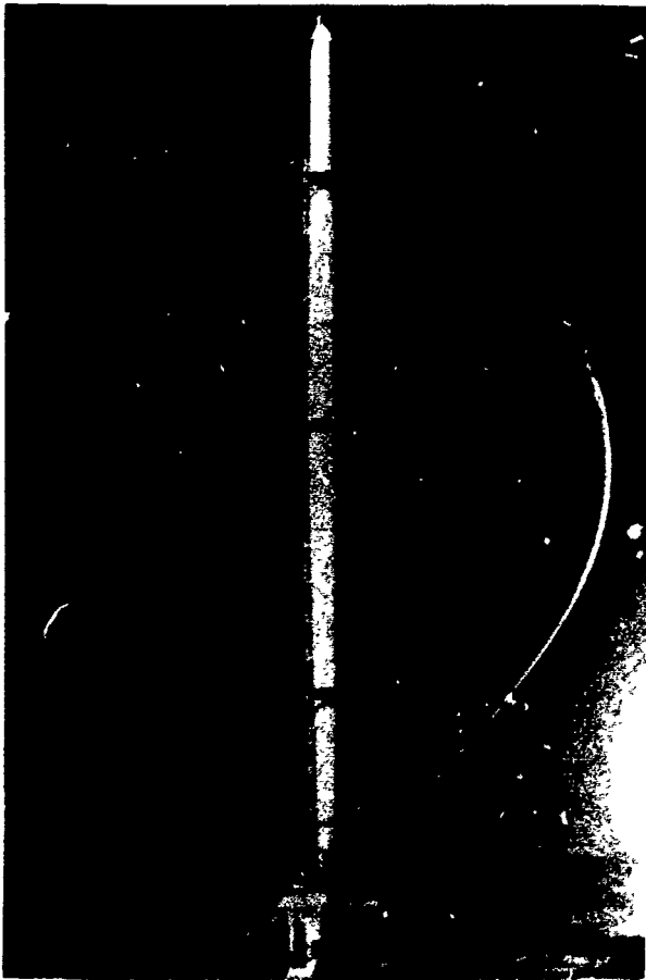
Figure 4-13.—A 500 kW Vertical-Axis Wind Turbine
