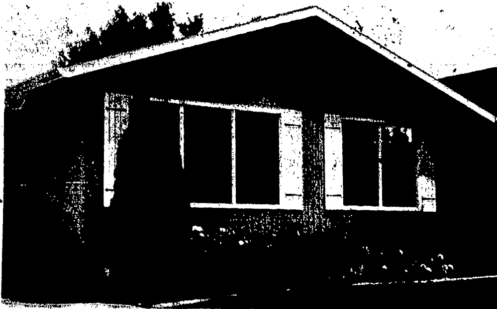
Before the Retrofit: R-8 walls Double glazing R-15 ceilings Yearly electrical usage: 40,062 kWh
