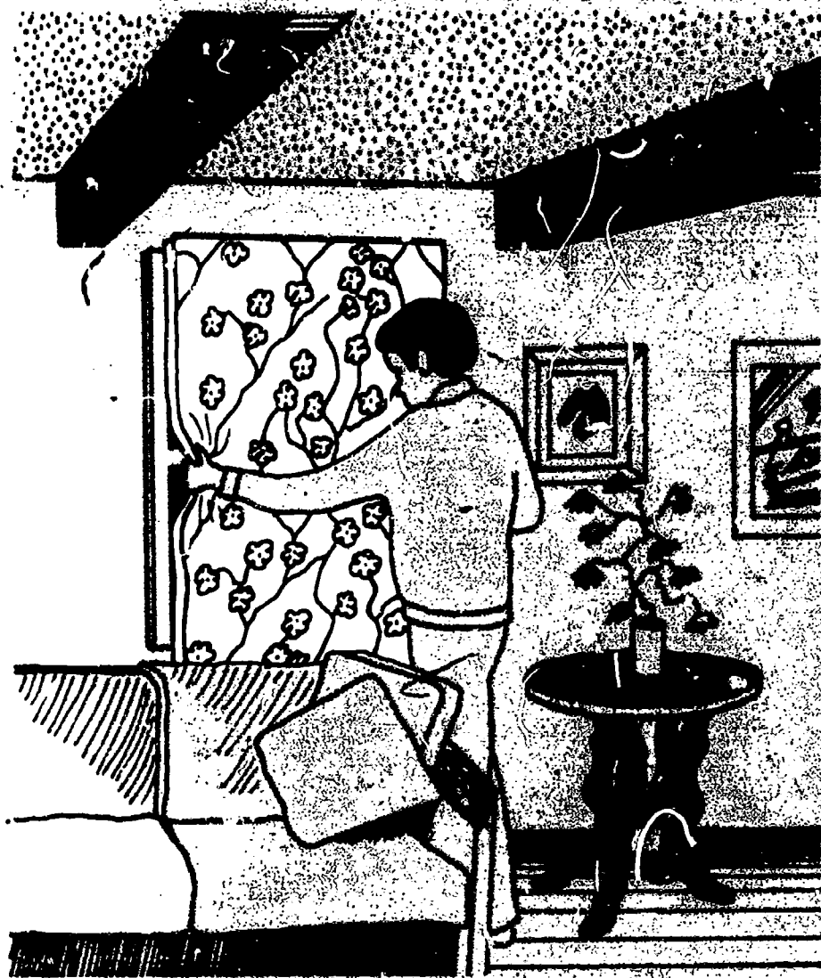
FIGURE 14: A pop-in panel is one of the easiest options for the do-it-yourselfer. Kits that include a flexible edge sealing system can help overcome the problem of out-of-square windows.
