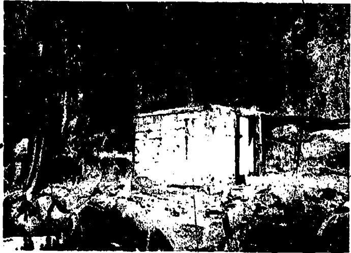
Vault containing recorders for seismic information in the Andes Mountains of northern Chile.
