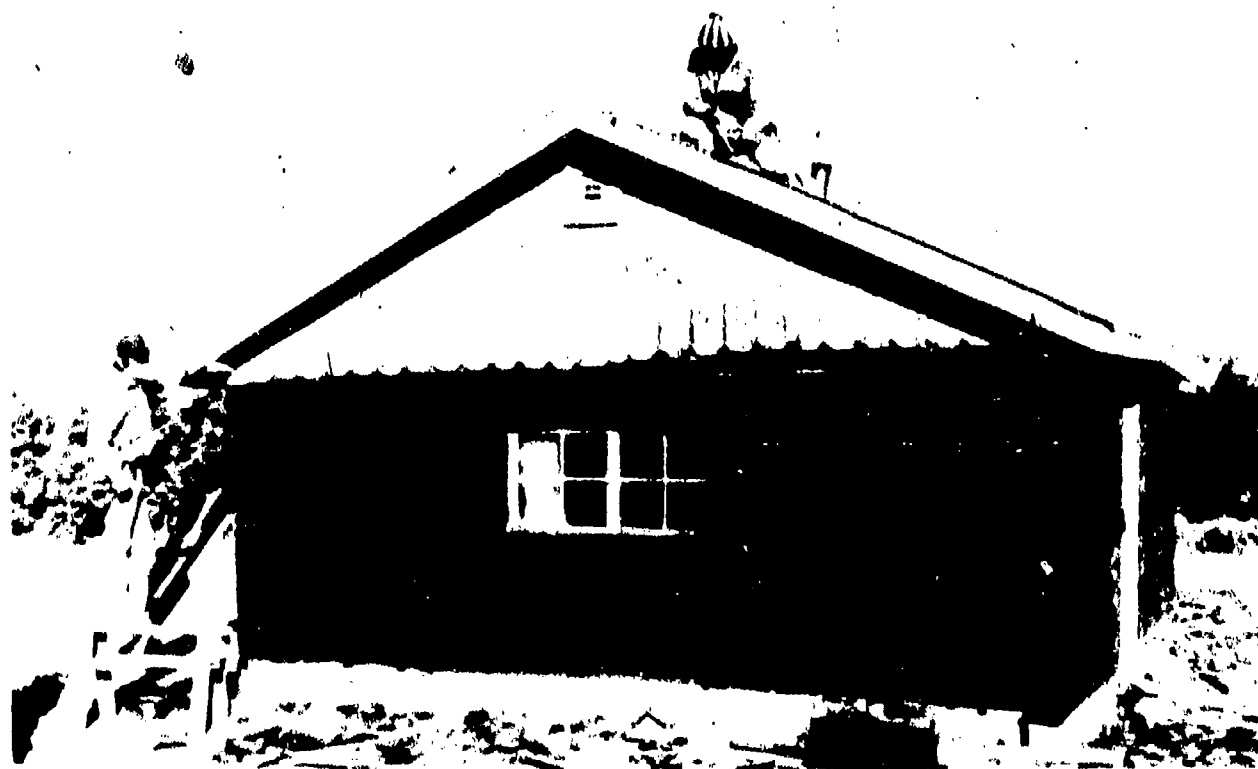
NPVTP giving on-site job construction experience.
