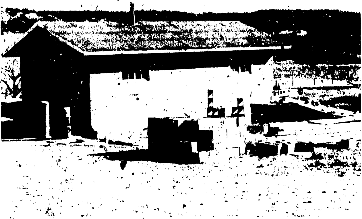
NPVTP Project scheduled to be completed with the aid of CETA labor. Cutbacks in the CETA funds has left four million dollars worth of material lay dormant with no labor to utilize them
