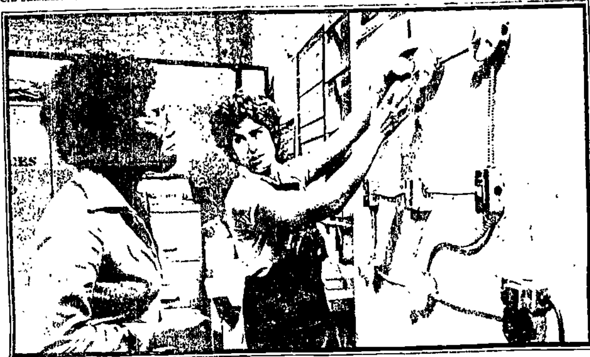
Cris Skidmore shows Jackie Breland how to bend electrical conduit.
