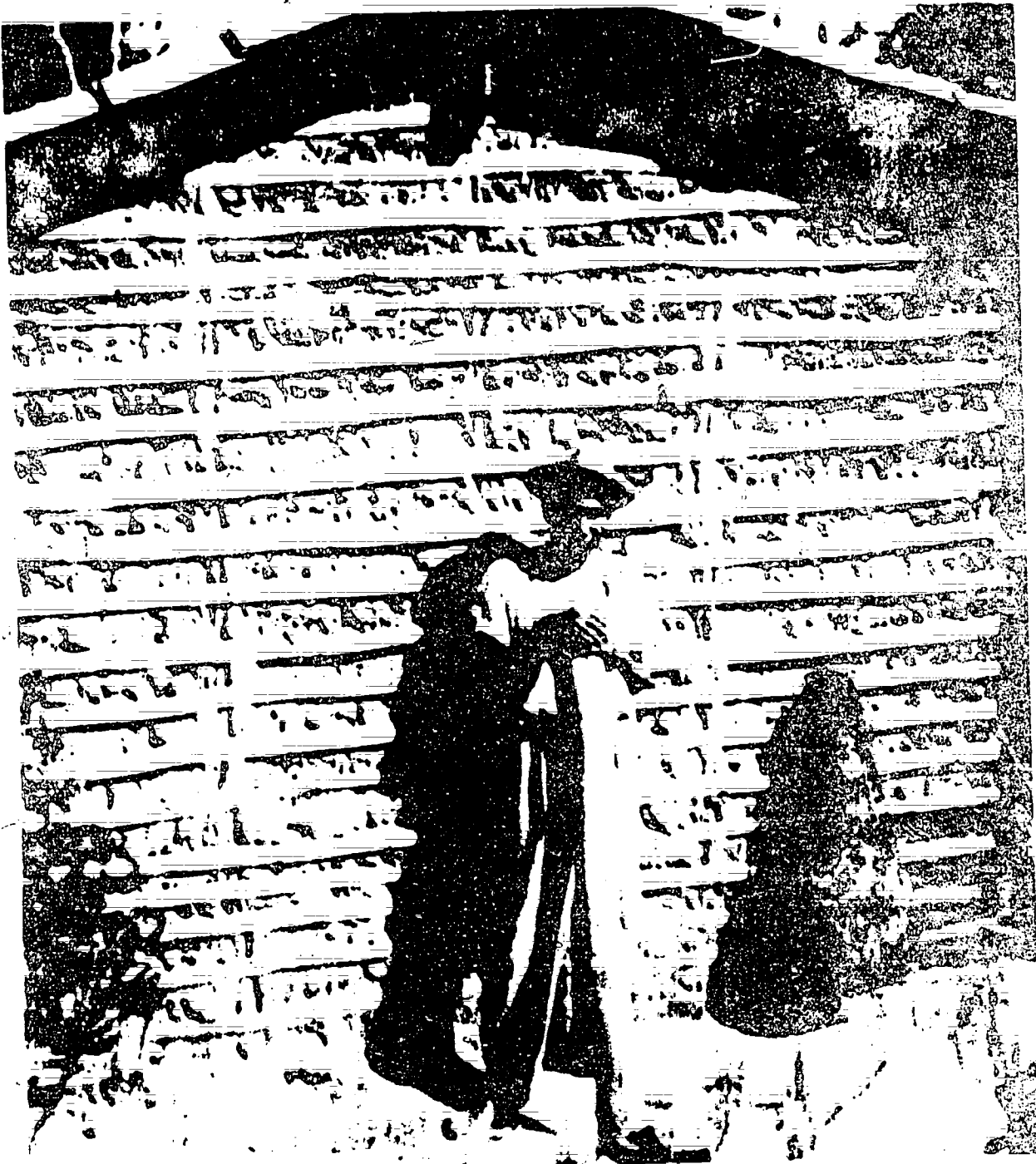
Figure 12:--Wide bamboo strips support and protect an adobe wall in El Salvador, forming a type of construction called bajareque in many Latin American countries. In El Salvador the common bamboo, Bambusa vulgaris , is available everywhere except in the driest areas, and its culms are standard material for many purposes.
