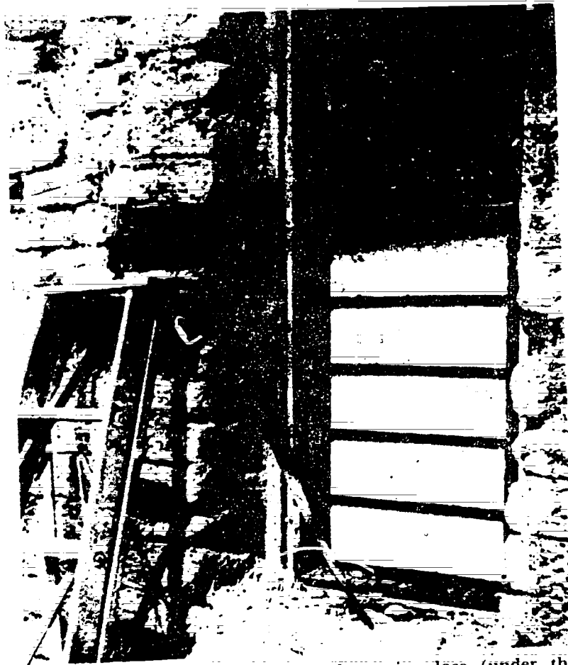
Figure 67b. The nailer block is shown in place (under the building paper) in this residence under construction in Albuquerque, N. M. (Koeber).
