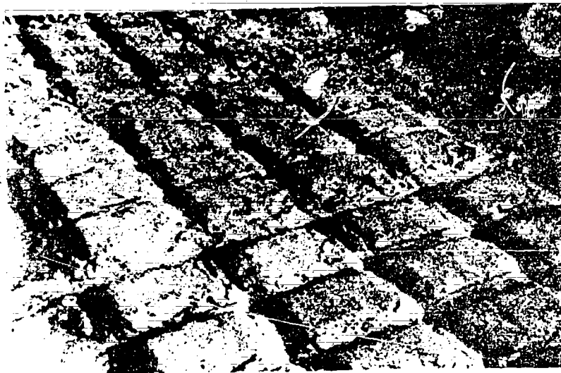
Figure 47. Inadequate protection of blocks during curing schedule may result in a loss such as occurred here after a rainstorm.
