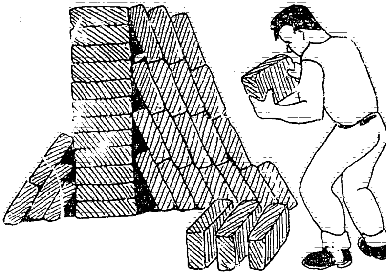
Figure 46. Adobe block is stacked after a month of curing.
