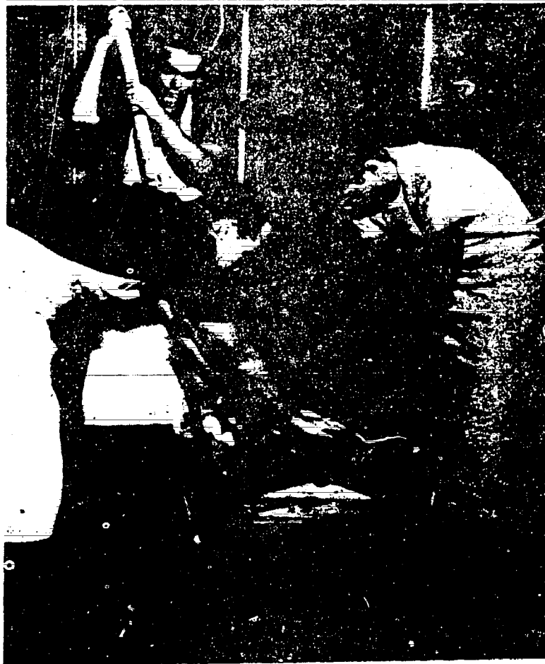
Figure 54. Charging mold box with soil mix.
