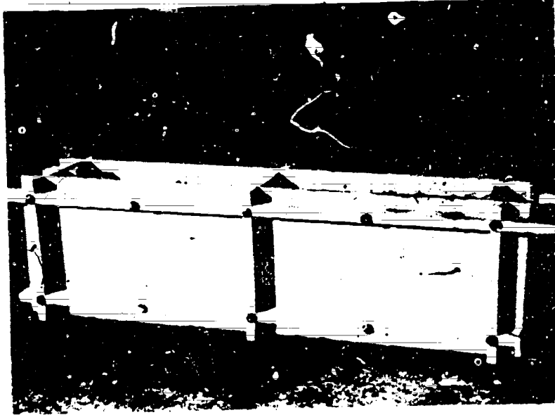
Figure 73. Straight form for rammed earth walls.
