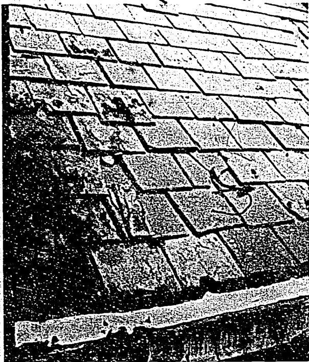
Renewal and replacement is now crucial for old and new campus building systems. Note damage on older slate roof (below), and newer flat roof (left).
