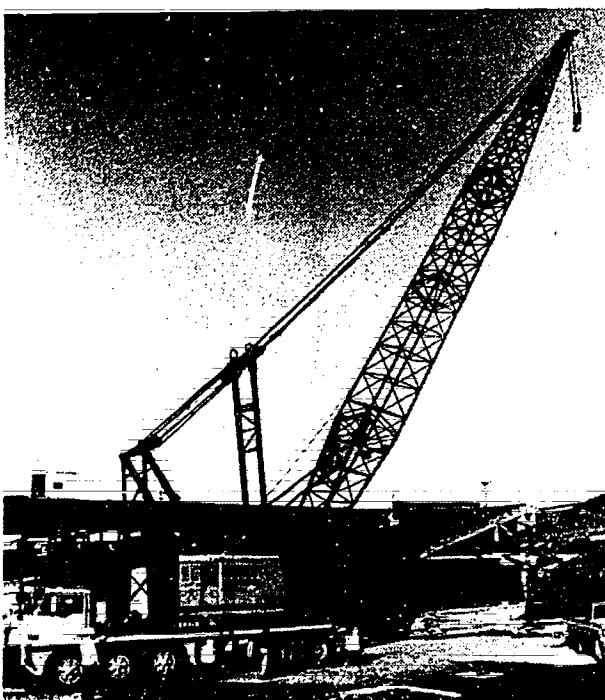
Figure 7-118. Boom Raised and Crane Moved to Area of Lift
