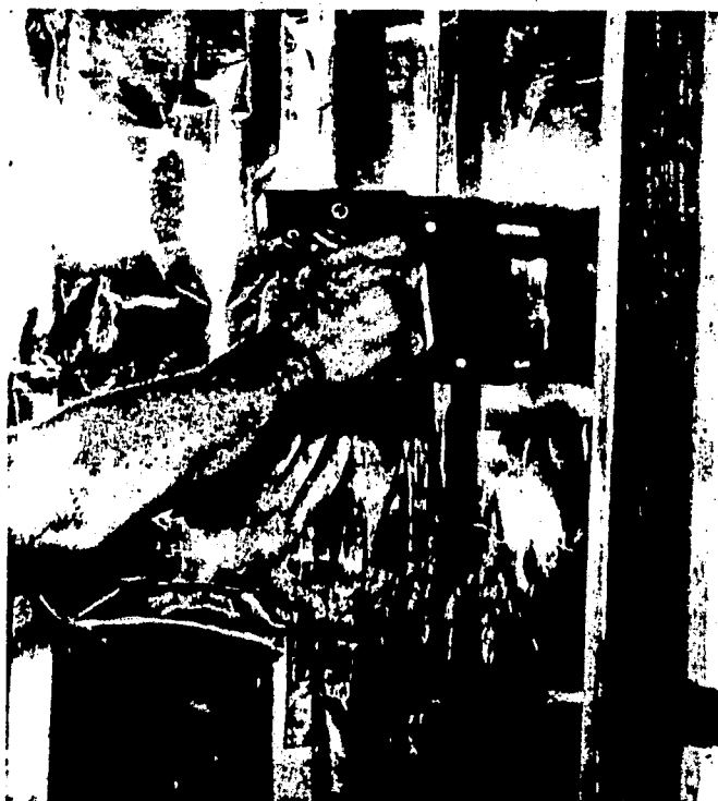
Fig. 13-25. Aluminum foil provides a good vapor barrier when joints are carefully lapped.
