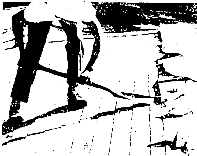
Fig. 10-24. Using a shovel to remove old asphalt shingles (Asphalt Roofing Manufacturers Assoc.)
