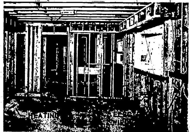
Fig. 13-4. Interior view of a residential structure with electrical, plumbing, and heating rough-in complete and ready for insulation materials.
