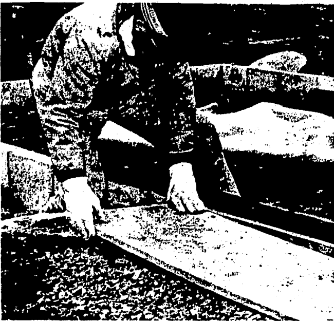
Fig. 13-45. Installing a rigid form of insulation in the perimeter of a slab floor. (Owens-Corning Fiberglas Corp.)
