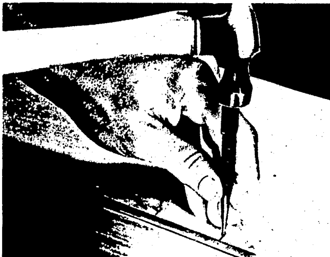
Fig. 8-9. Setting a nail.
