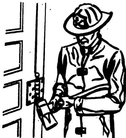
Figure 14. Removing Hinge Pins.
