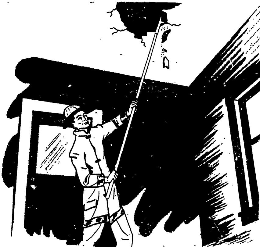
Figure 22. Removing Plastered Ceiling.
