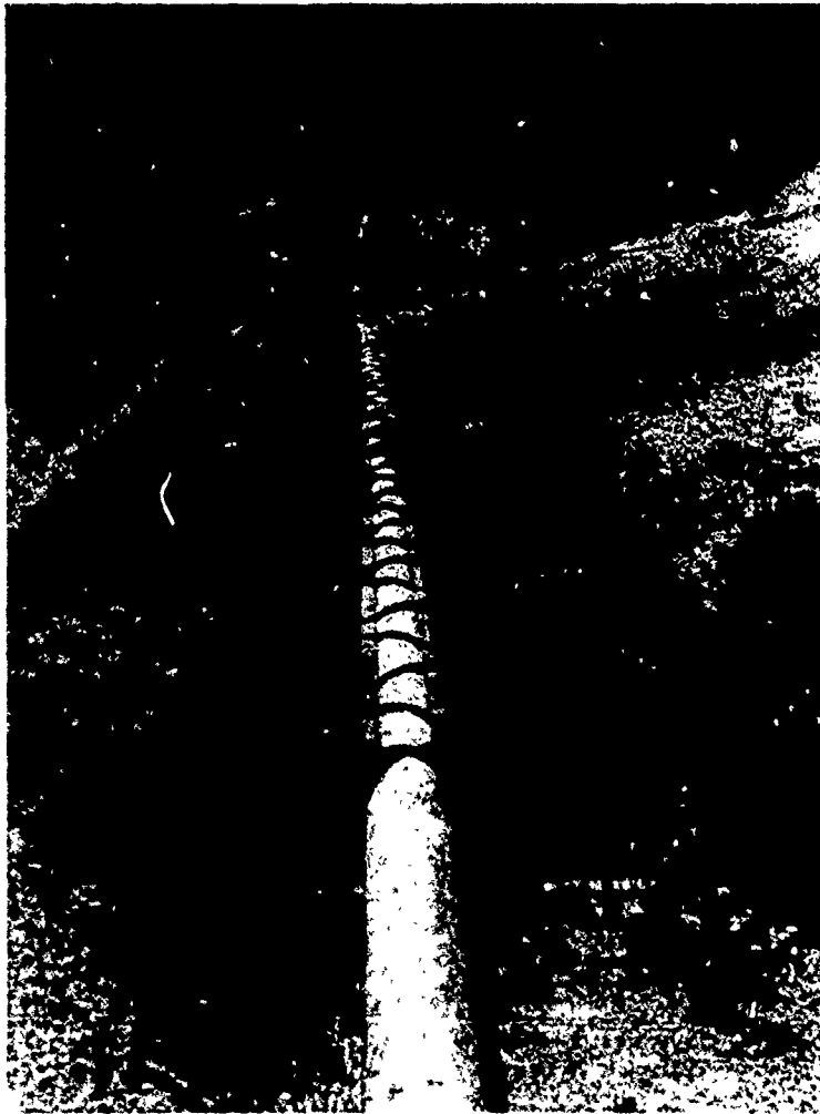
FIG. 28 Water pipeline, normally underground, rests on ground surface where, encased in protective steel sleeve, it crosses an active mudflow.
