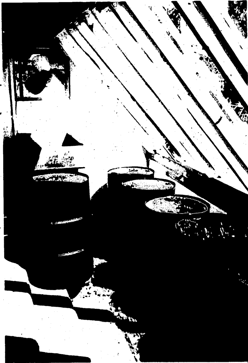
Barrels filled with water support plant beds (under construction) and collect solar heat by day, then release the heat at night. Since no shade cloth is used, the fan is necessary to ventilate the greenhouse in summer. (Strandquist Greenhouse, Berryville)
