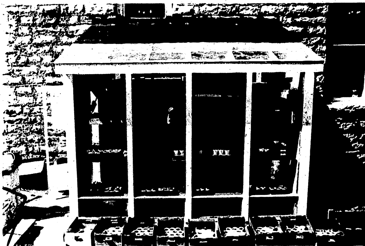
Bill Brown of the Office of Human Concern designed this vertical glazed solar greenhouse for the senior center in Berryville. Half of the roof is glazed with fiberglass to permit light to enter from above and permit a light balance within the greenhouse. A row of vents along the bottom of the south glazing and side wall vents provide ventilation. There are four levels of plant shelves, each one supported by the vertical glazing columns. The senior center profitably sells plants and vegetables to residents of the community. (Photo by Bill Brown).
