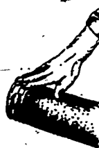
LUBRICANT IS APPLIED TO SPIGOT END
