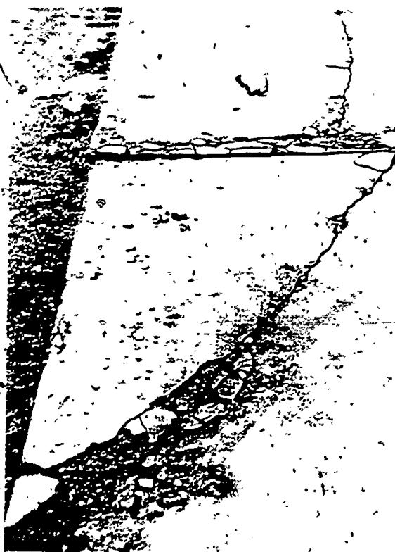
Figure 1-8. Effect of frost heave on rigid pavement.
