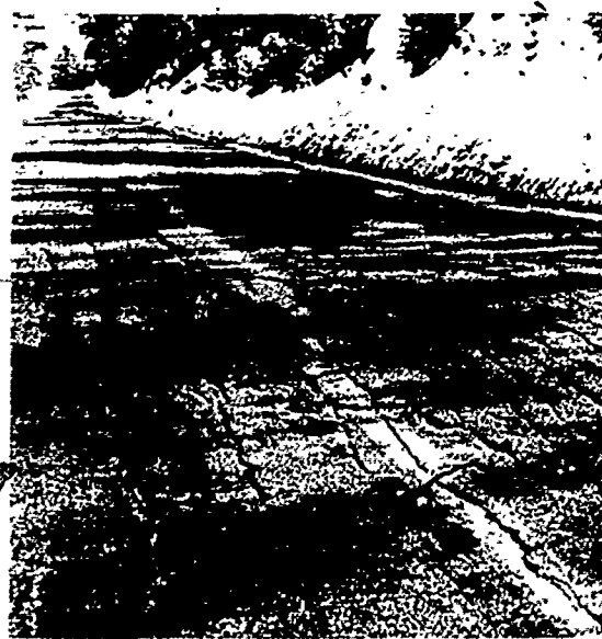
Figure 1-7. Effect of frost heave on flexible pavement.
