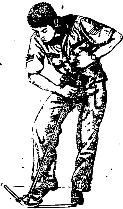
Figure 31. Floor Bend With EMT™
