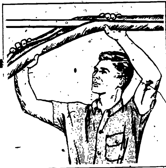
Figure 4-11. Installing flex rubber insulation.
