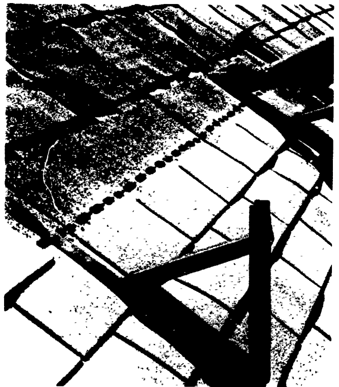
Fig. 8-18. Roof bracket for 2" x 6" plank
