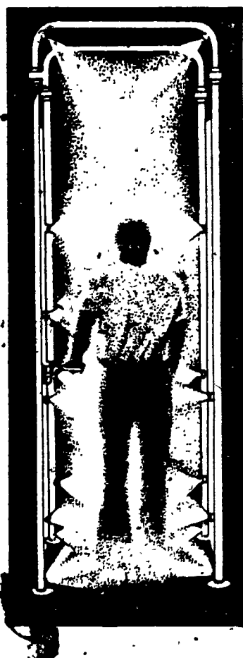
Figure 6. Emergency safety shower - eye wash.
