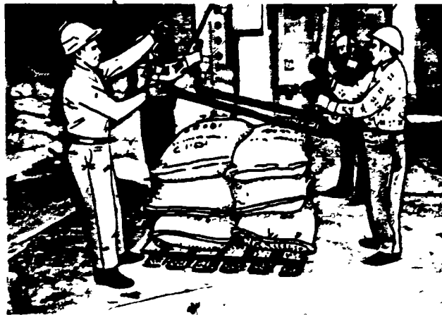
Figure 11. Wing pallet is loaded on to bar bridle.
