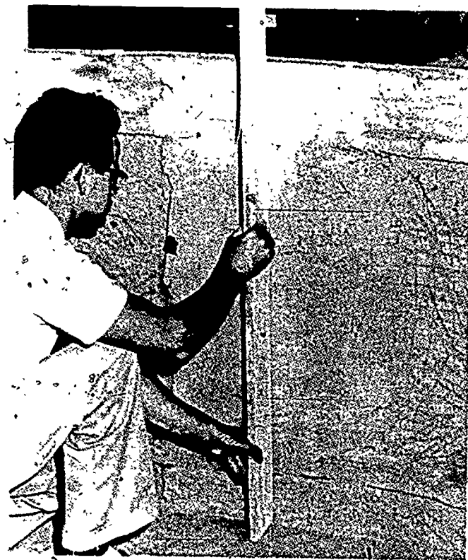
Fig. E-91. Checking plumb with a straightedge.
