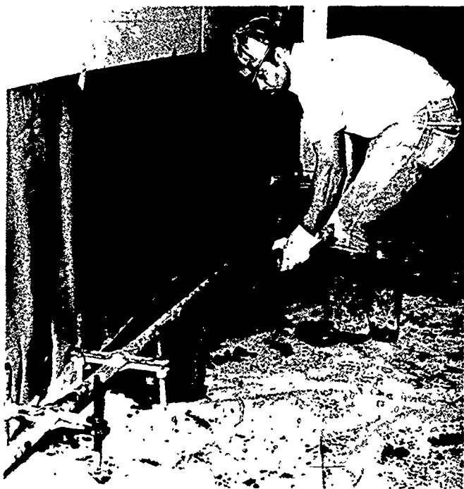
Fig. E-2. Forming the setting bed
