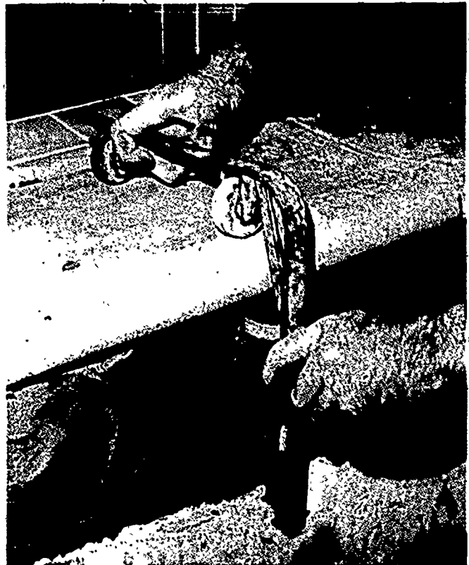
Fig. E-118. Floating the mortar with a roller-skate template
