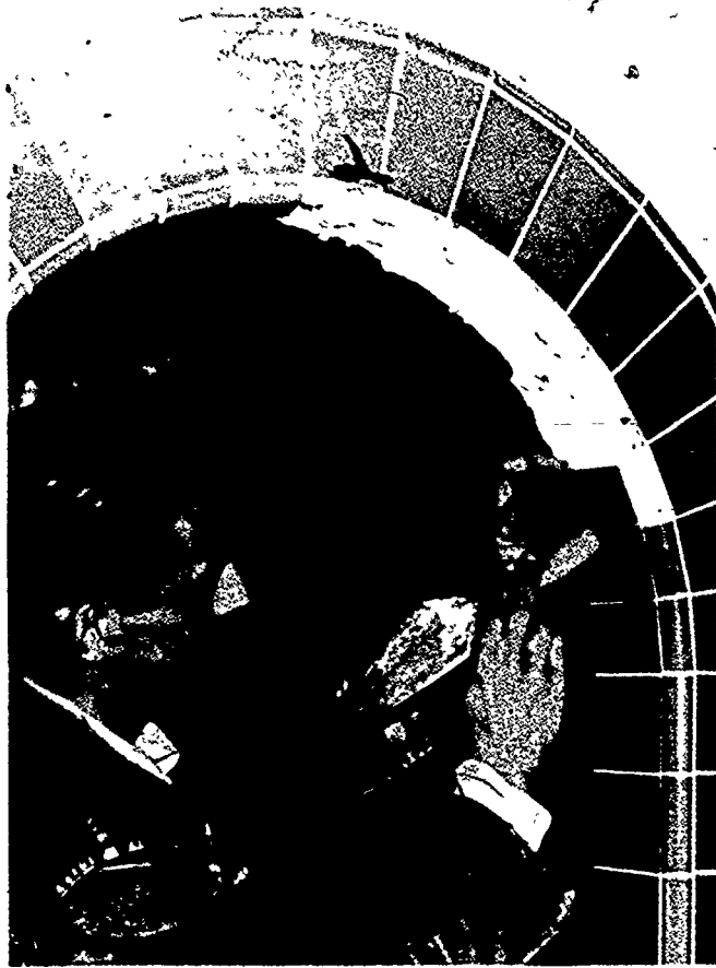
Fig. E-76. Setting tile on intrados of arch
