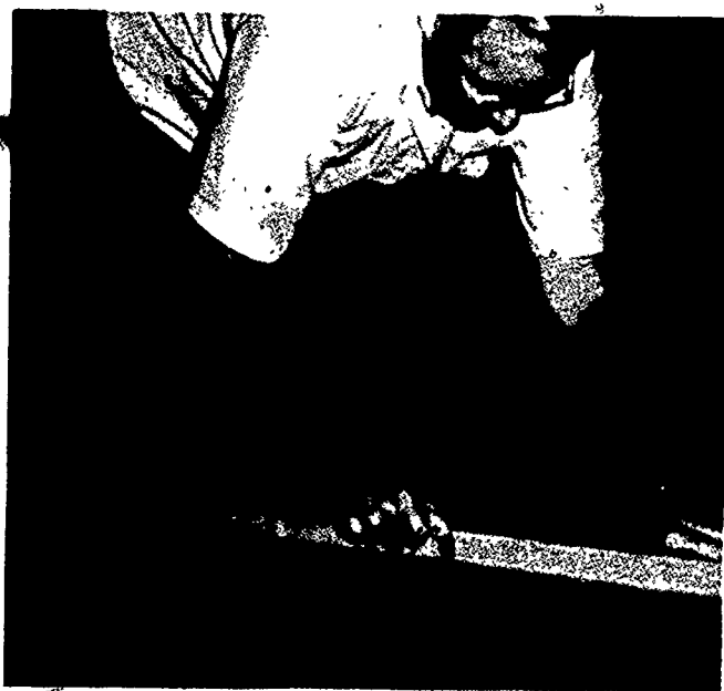
Fig. D-16. Scoring of glass fiber board with scoring tool and straightedge
