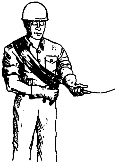
Figure 7-22.—Carrying tie wire.
