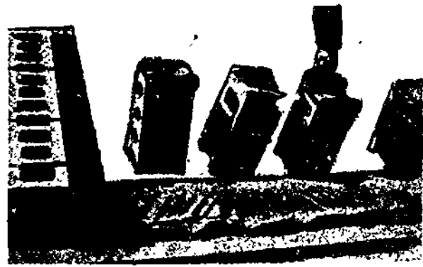
Figure 8-13.—Blocks buttered for vertical joints.
