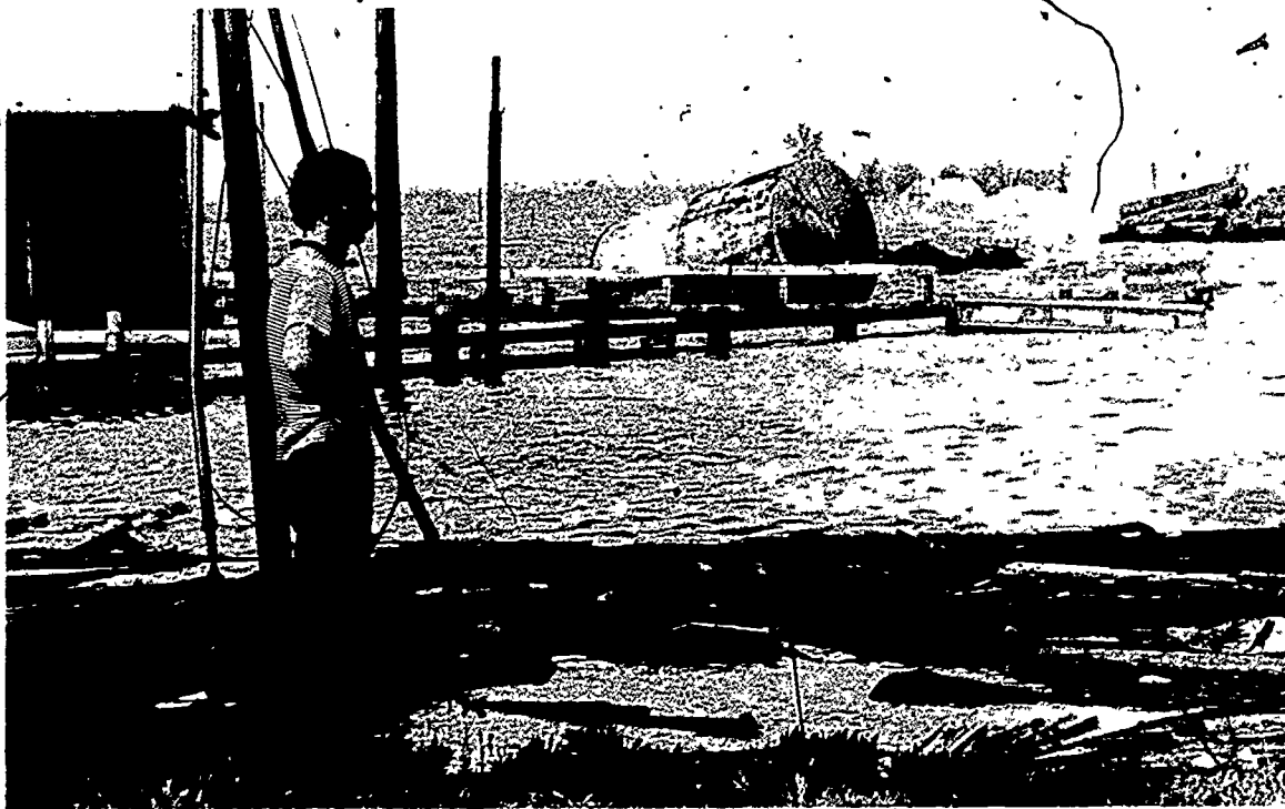
VISTA volunteer in St. Louis area surveys damage caused by flood.
