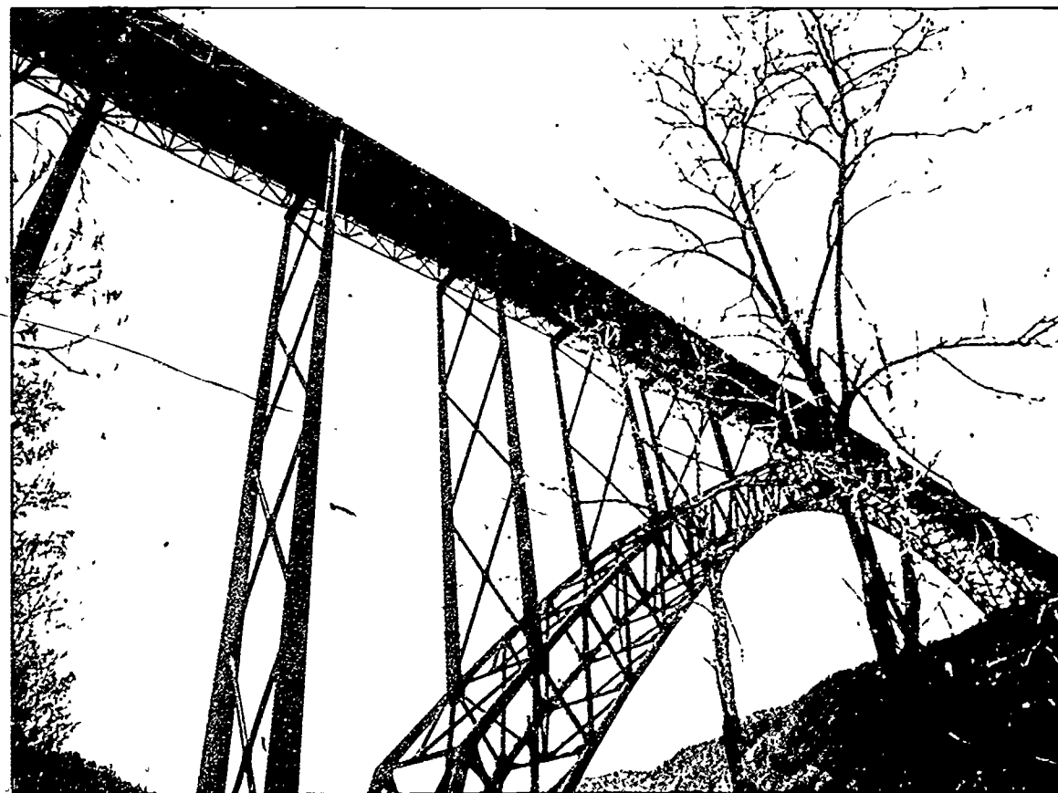
The New River bridge in Fayette County, West Virginia, completed in 1977, is the largest single road project of the Appalachian Development Highway System.
