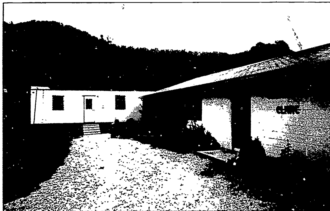
The ARC-funded Clear Fork Clinic in Clairfield, Tennessee, is equipped to provide dental services as well as primary health care.
