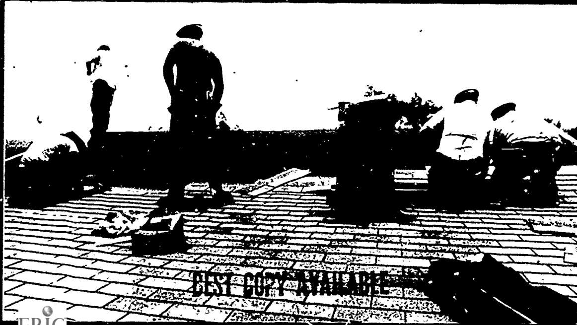
(TOP LEFT) In Cumberland, the labor-management committee has succeeded in nipping potential problems in the bud. (LEFT) The repair and re-roofing crews are putting a new roof on an Allegheny County house under the housing rehabilitation program.
