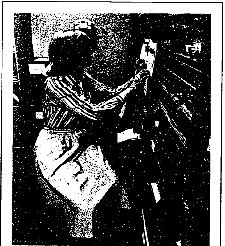
Edna is proud of the station's equipment, much of which she installed herself. "I have to keep checking it to make sure everything works right."
