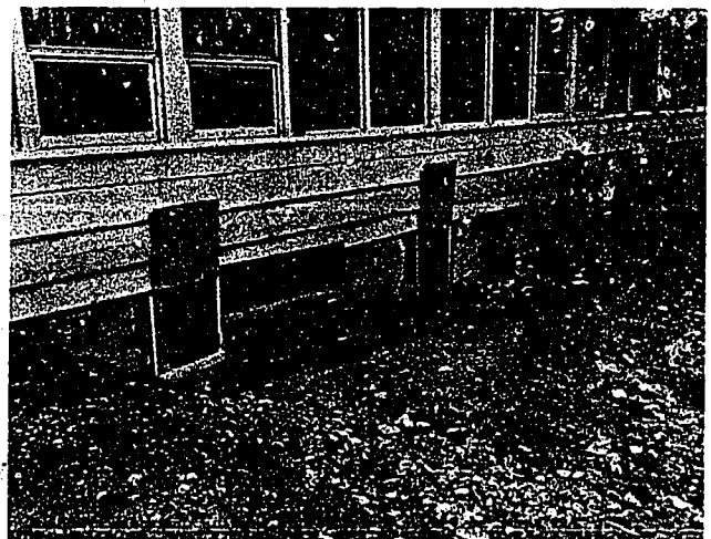
Figure 40. School house built on permafrost in Glenallen, Alaska in 1953. Air vents in foundation are opened in winter to allow cold air circulation between floor and ground and are closed in summer when school is not heated. The jacks allow correction if any heaving or settling occurs. (Photo No. 915, by Troy L. Pêwé, Arizona State University.)
