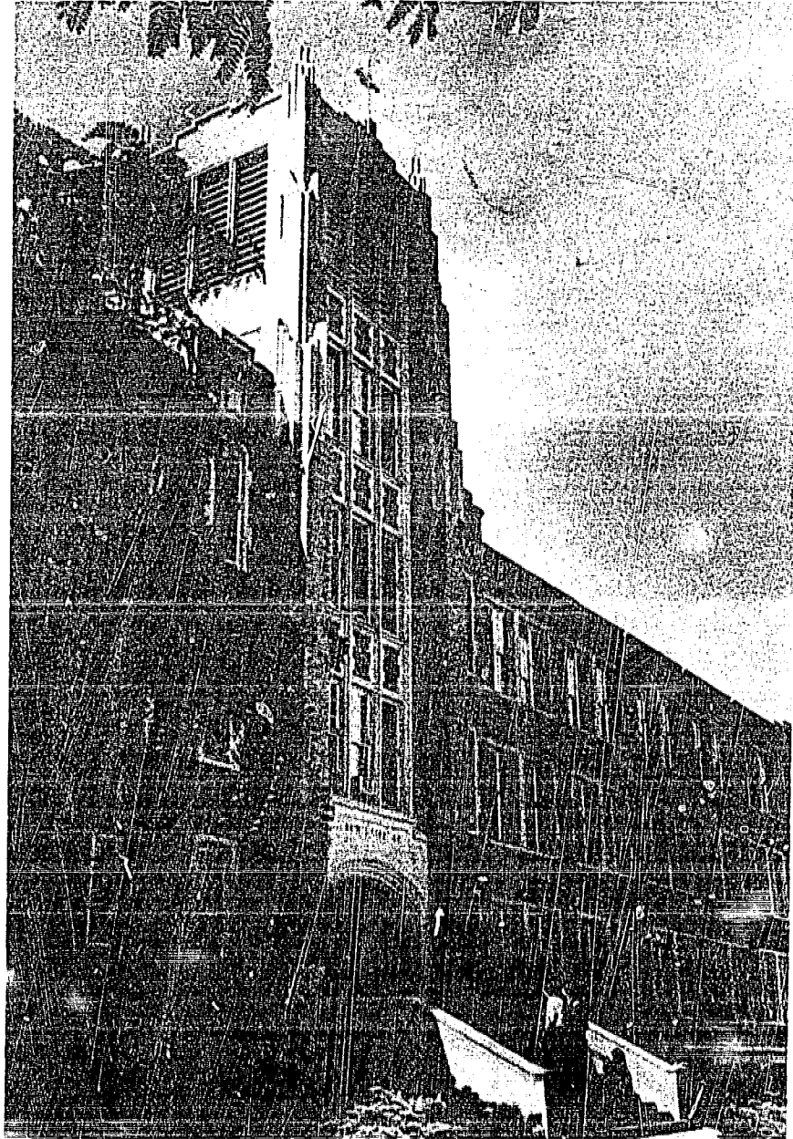
The Aquinas College Administration Building
